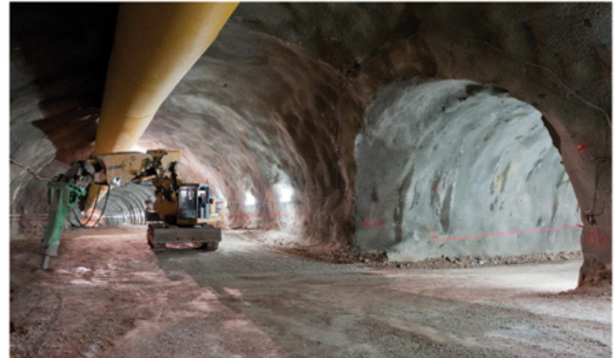
Autoroute Corinthe-Patras Tunnels Panagopoula
